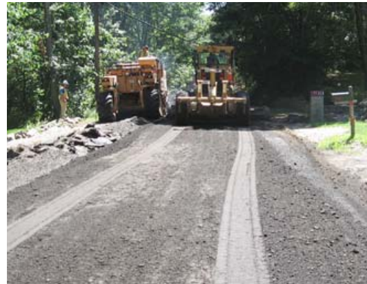
Reclaimed section being graded
