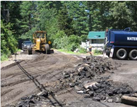
Atkinson Road intersection being reclaimed
