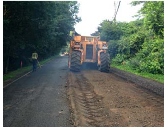
Pavement reclamation grading operation
