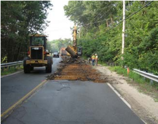
Busby construction begins pavement reclamation over Spicket River
